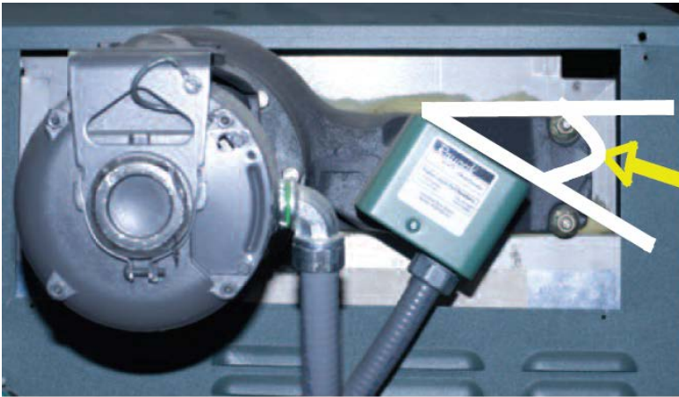
RAYTHERM Models 514-1826 with Integral Pump Flow switch must be tilted 25^{\circ} \pm 5^{\circ} From Horizontal Figure 7
